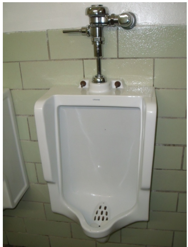
This 1.0 gallon per flush urinal fixture is the current urinal fixture of choice in the building.
