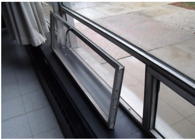
Many of the windows in the building have aged over time, some becoming inoperable. In this picture one inoperable window is shown.
