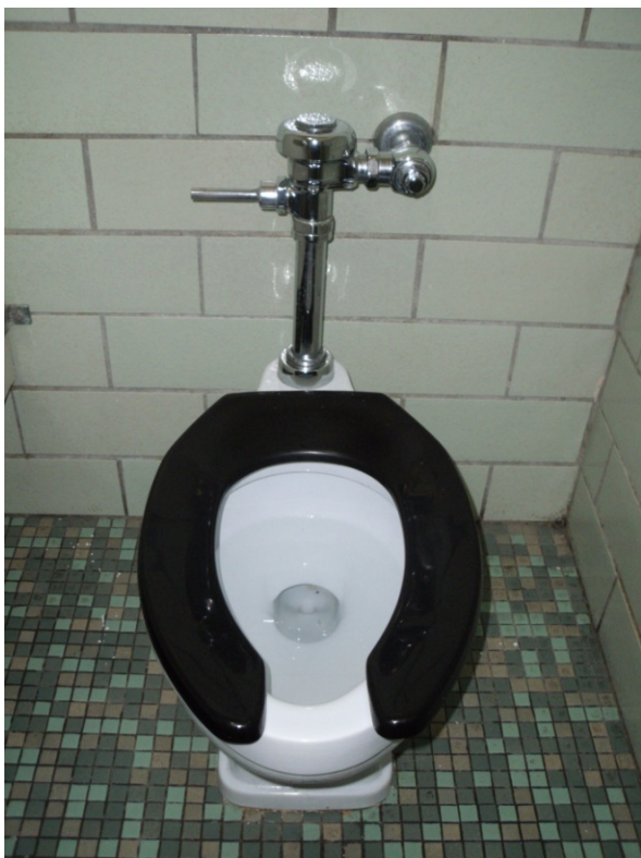
View of current toilet fixture found throughout the DTD house. All toilets found throughout the house use 3.5 gallons per flush.
