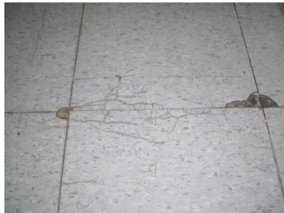
There are several areas in the building where tile is used to cover the floor. After many years of wear and tear the existing tile floor has begun to chip and crack way as pictued above.
