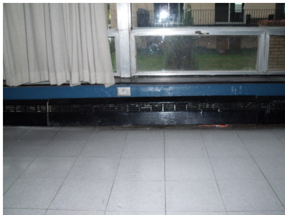
Picture viewing one of the many runs of raditors that around found throughout the building.
