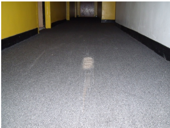
Exsiting run of carpet found in the upstairs hallway of the Delta Tau Delta chapter house. Note of the wear of the carpet in the center of the photo.
