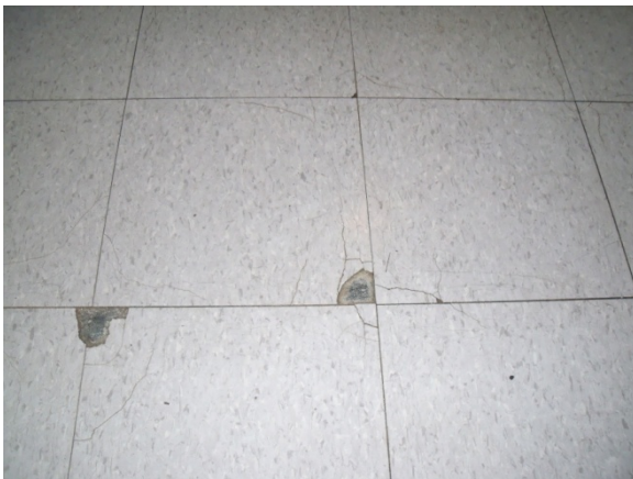
There are several areas in the building where tile is used to cover the floor. After many years of wear and tear the existing tile floor has begun to chip and crack way as pictued above.
