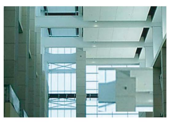
In the main exhibition hall, due to a large amount of space that needed to be controlled, a combination of draft curtains and ceiling smoke and heat vents were used. The draft curtains act as a physical barrier that contains and directs smoke flow in the event of a fire, while the vents exhaust the smoke out of the building.
