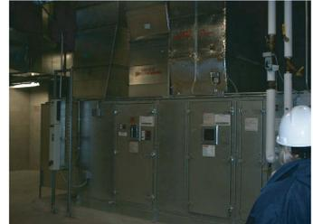
The McCormick Place smoke control system is integrated with the HVAC system. The building area is divided to a certain number of zones. Each zone is served by a number of air handling units. In case of fire, the air handling units of the area affected will switch to exhaust mode in order to keep the egress space free from smoke for the time of evacuation.
