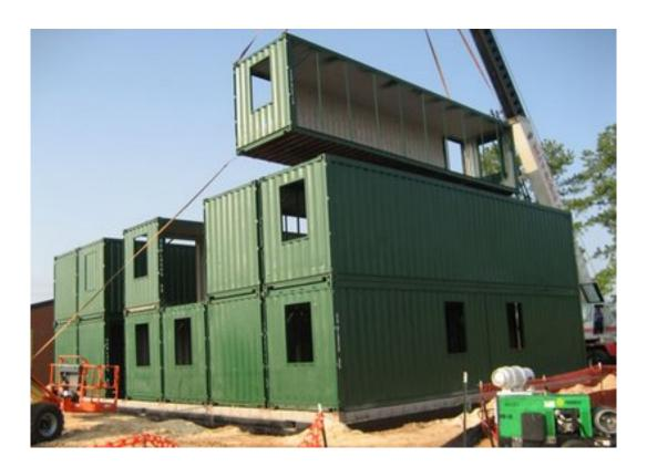
The Full Scale Model group worked to create and construct the site plan for the full scale model that would stimulate support and exposure in the community as well city-wide. The full scale model would be used to showcase the advantages to this method of constructing houses and serve as a tangible example of the soundness of this idea.
