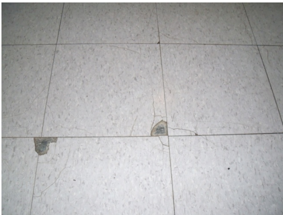
There are several areas in the building where tile is used to cover the floor. After many years of wear and tear the existing tile floor has begun to chip and crack way as pictured above.
