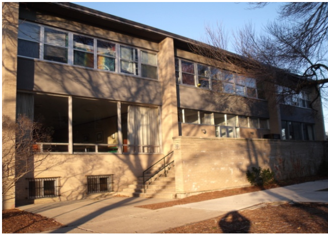
Delta Tau Delta – Windows on the south side of the building
