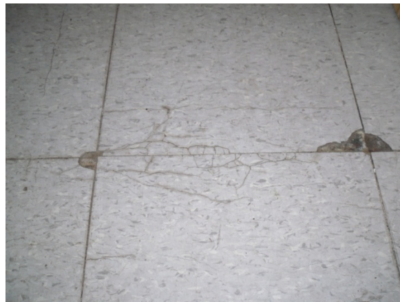
There are several areas in the building where tile is used to cover the floor. After many years of wear and tear the existing tile floor has begun to chip and crack way as pictured above.
