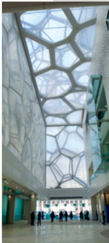
ETFE Skylight / Facade translucent Inflatable cushions low U-value printed PV cells
