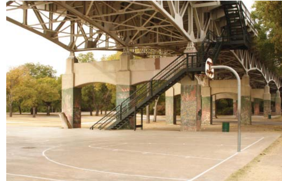
Adapted space below bridge
