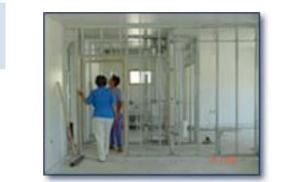
Interior non-load bearing walls can now be built with wood or steel studs and drywall.
