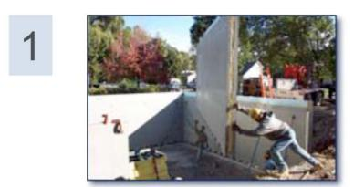
Prefabricated panels are brought to the site by trucks and put in place by cranes.
