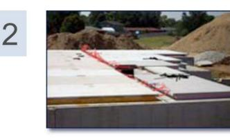
Floor panels are put in place after a wall level is in place.
