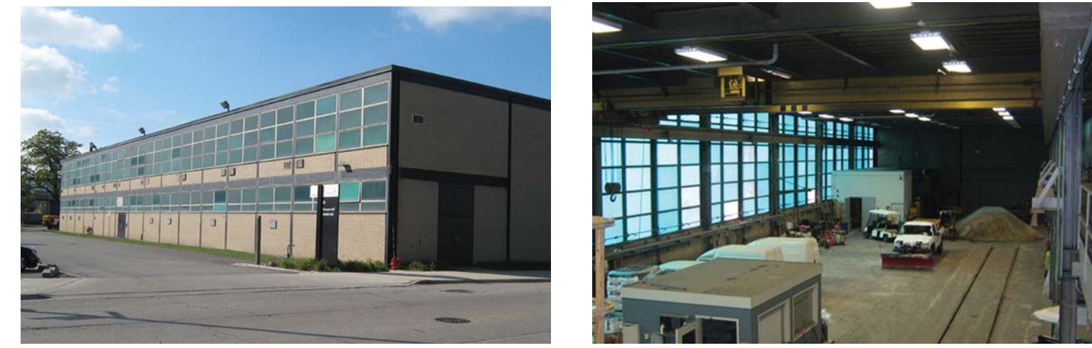
The existing facility is a steel structure with a brick and glass enclosure. It currently holds maintenance and landscaping equipment.
