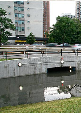
When the combined sewer overflows the water can come back out of inlets and drains causing flooding.
