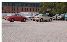
Permeable paving used for parking lots and sidewalks to help with storm retention
