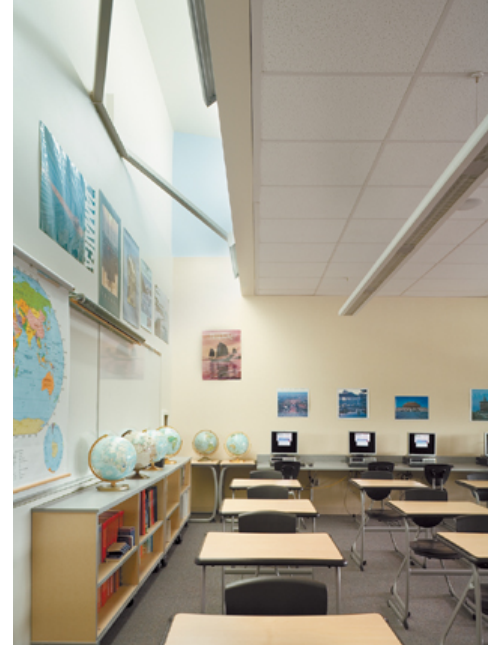
Classroom Natural Lighting Shaft
