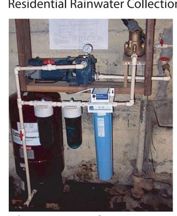
Filtering system for Rainwater
