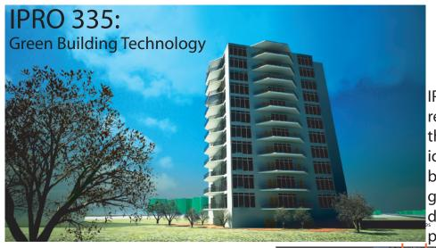
IPRO 335 designed student housing to replace Gunsalas Hall on the IIT Campus. In the design we aspired to incorporate green ideals. In the new design we used green building technologies such as a green roof, grey water recycling, PV solar panels, double facade, chimney affect, and native plantings.
