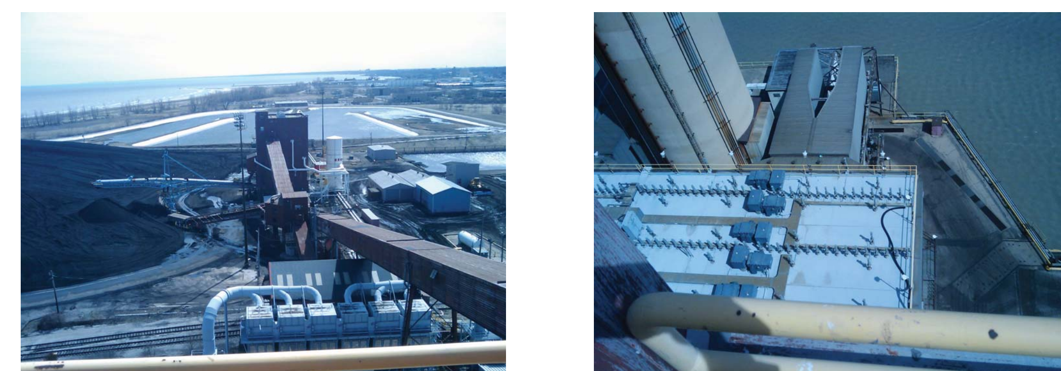
photos from Waukegan power plant visit
