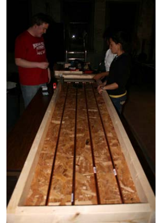
Solar Collector Prior to Aluminum Sheets being installed
