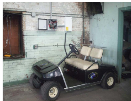
End Product after installation and
