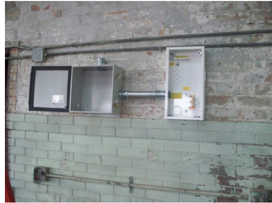
System Prior to installation
