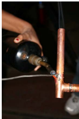
Soldering of the copper pipes
