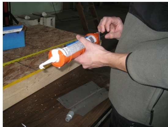
Caulk was used for fastening the wood to itself
