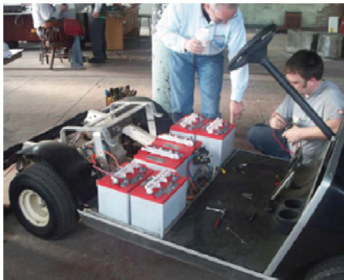
Installation and Connection of Battery Bank
