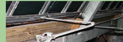
Figure 2: Current roof window system in Machinery Hall.
