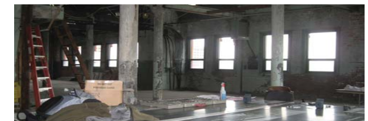
Fourth Floor Machinery Hall - Zero Energy Lab
