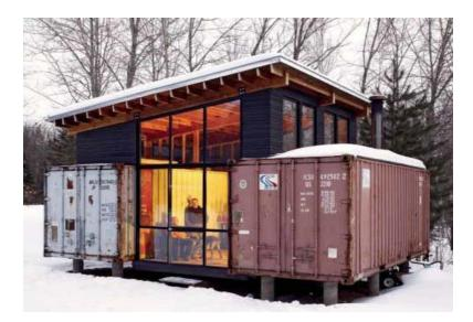
A modular building, similar to prefab, would be designed and built off site. However, the modular building would arrive at the final destination as one unit rather than a kit of part. For example, a recycled shipping container could function as structure and enclosure.
