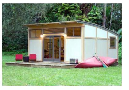
Prefab buildings are built off site, shipped to the final location by various means and assembled on a prepared site as a kit of parts
