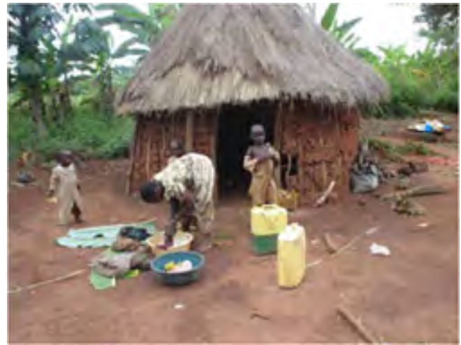
Traditional mud/stick construction with thatched roof.
