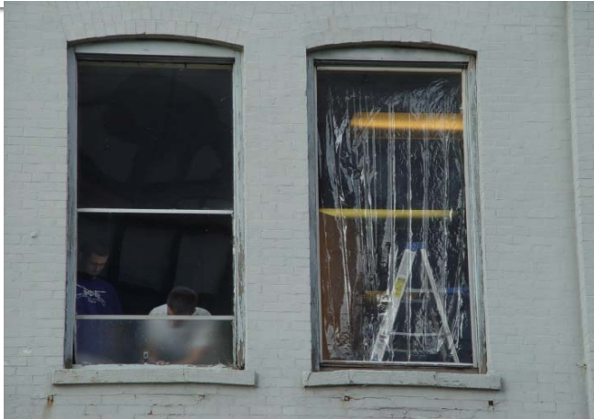
Installation of window film
