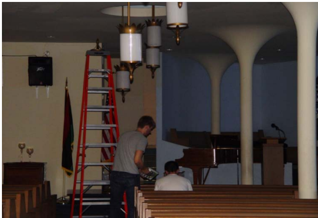
Changing out light fixtures
