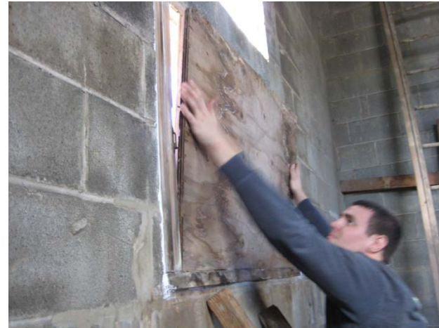
Insulating hole in steeple
