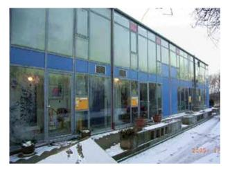
The Northern part of the Passive House in Darmstadt Kranichstein has a spacious glazed space, which is not heated. There are only single pane windows used - during frost there will be frost patterns on the panes. A splendid example is shown in the next image. In the image above the fresh air inlets in a height of 2.80 m can be seen.
