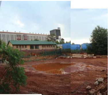
internal site view south
