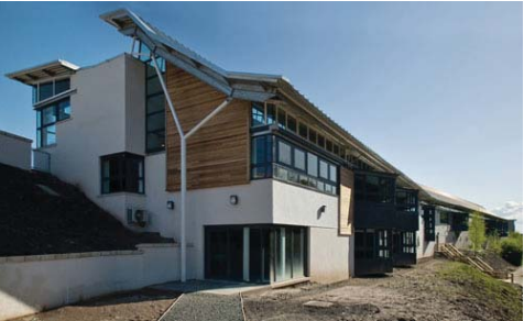
Approach and corner view along the river.
