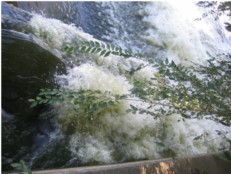
Fig. 22. Fish ladder at Elgin Dam.
