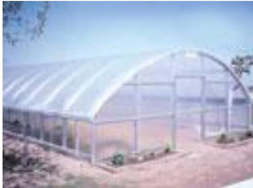
Figure 1 Cold Form Greenhouse Structure
