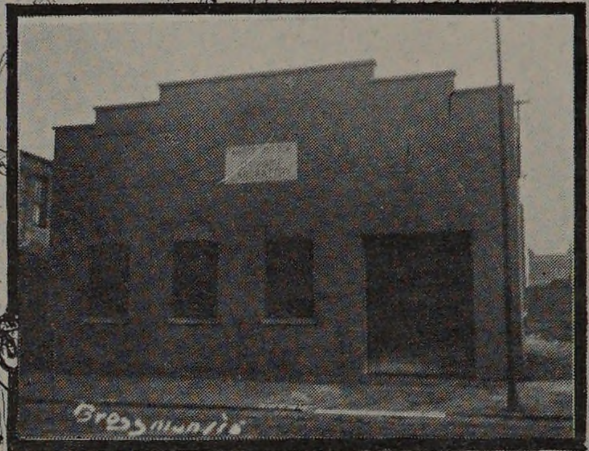
TESTING-LABORATORY & ICE PLANT
