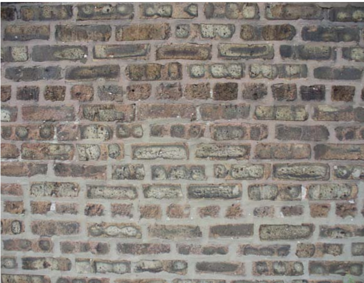
masonry common bond
