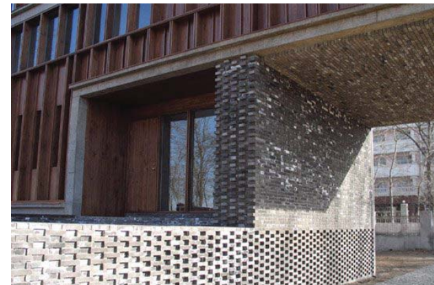
Tongxian Gatehouse Office dA Beijing, China
