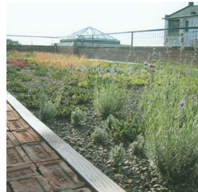
Bricks as green roof pavers Benton Brown Loft conversion, NY
