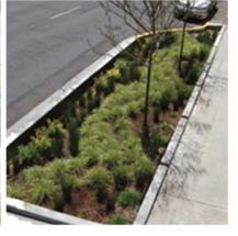
Curb Extension: Extend out into the street to provide a location for vegetation to capture rainwater. Can also integrate bike paths and pedestrian crossings
