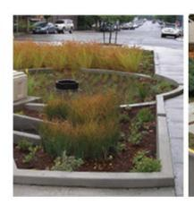
Rain Garden: For locations with ample space. Can also be used to soften or adjust intersections that are unsafe for pedestrians or cyclists.
