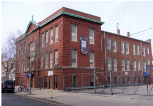
Site: Erie Elementary Charter School - located in the former parochial school of St. Mark Roman Catholic Church in the SE corner of Humboldt Park neighborhood of Chicago.
