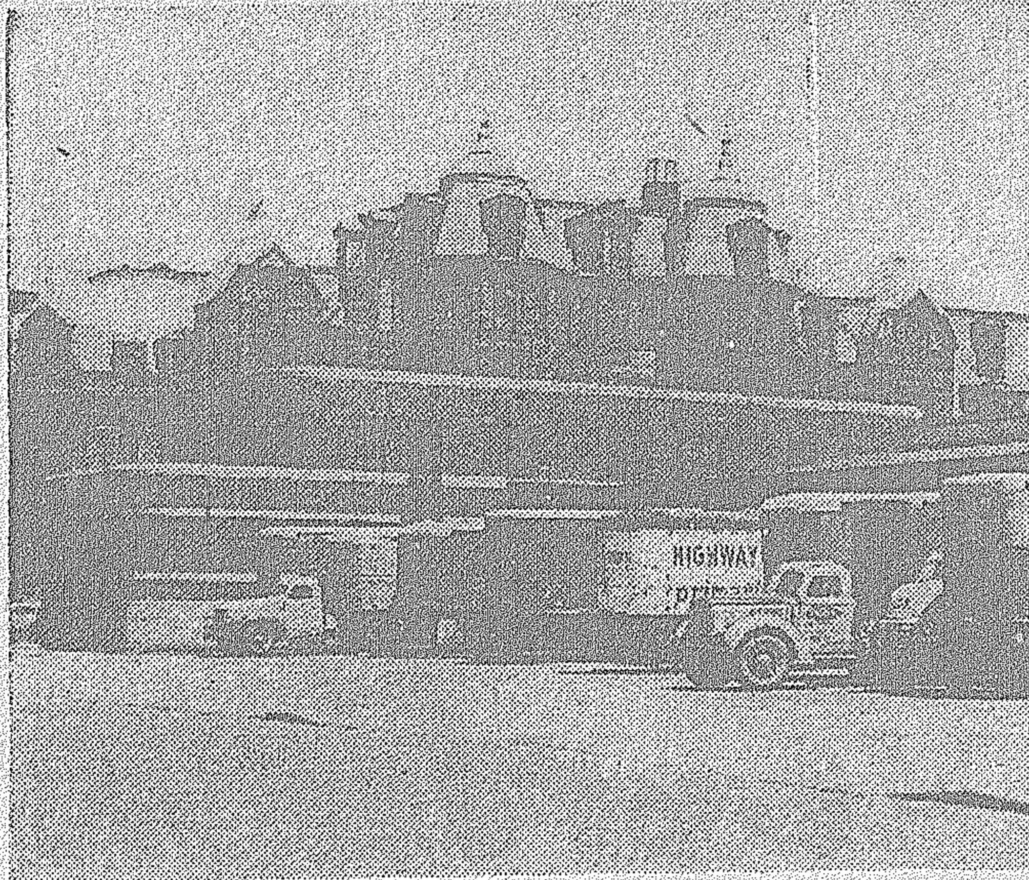
THE LATEST ADDITION to the new Technology Center area is the Huber and Huber trucking company property at 33rd and Wabash. The 50,000 square foot area, for which contract arrangements are being made, will be occupied by the Institute as soon as the company moves to its new location on the southwest side of the city.
