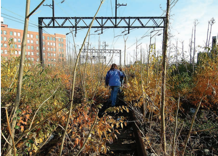
Reading Viaduct Philadelphia, PA
