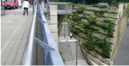
Planted stair entrance
