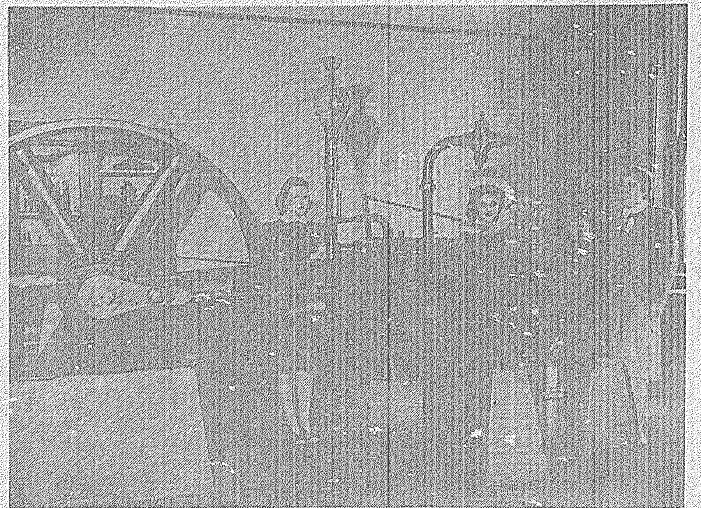
What do I do now? No kidding, these girls really know what this Corliss one lugger is all about. Alda takes the RPM reading with a tachometer, Mercedes throws in the governor control, Dorothy opens the throttle valve, and group leader Lillian keeps check on the steam pressure. After a test run with constant load conditions, they put their heads together and come out with an efficiency of 78.1%.
