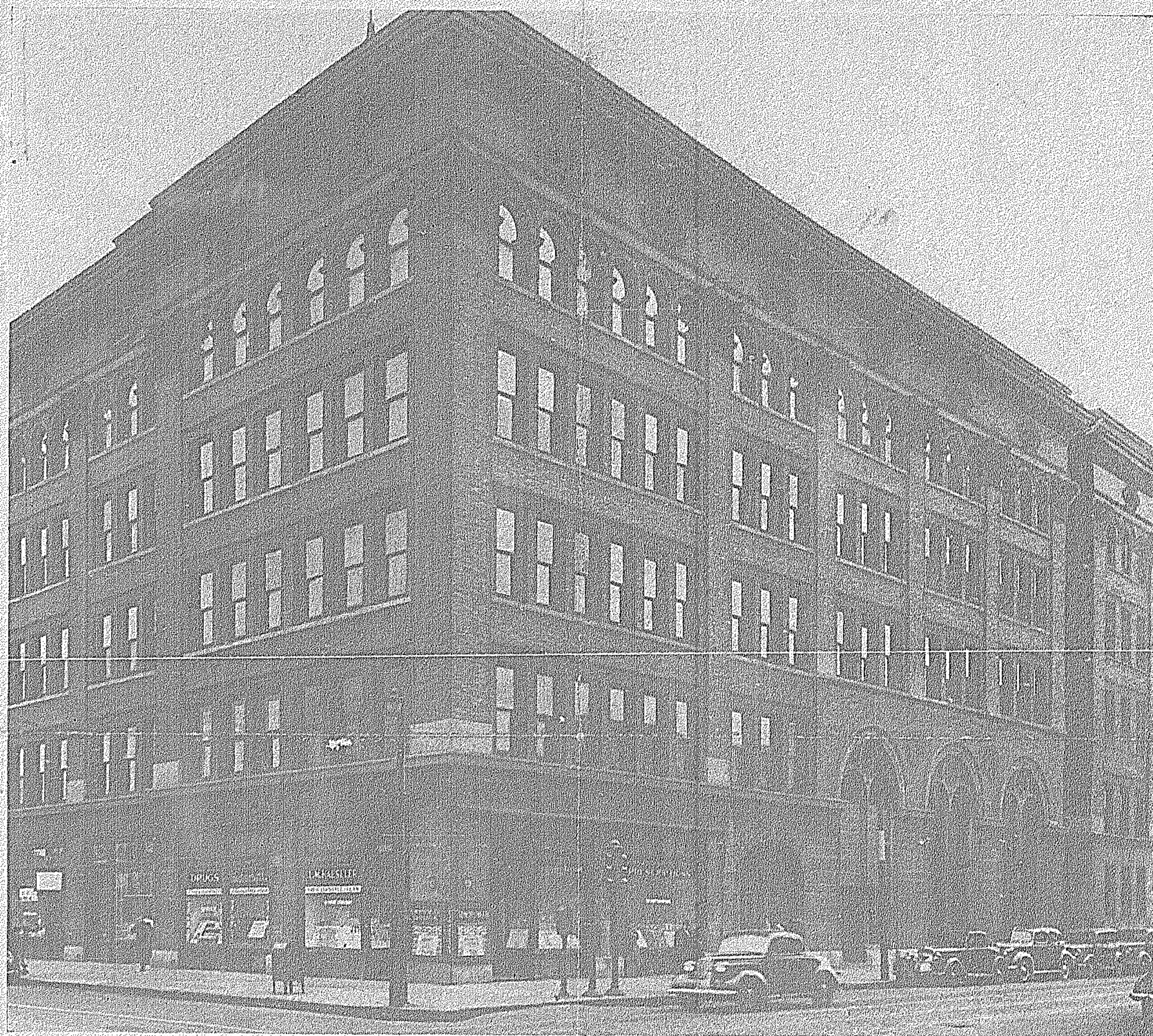
View of Main Building of Lewis Institute. Building is located at 1951 W. Madison Street and houses curriculum including pre-professional, engineering, and liberal arts courses.
